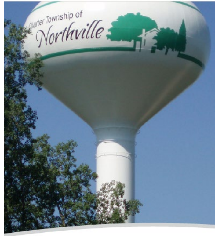
Waterspheroid® ELEVATED WATER STORAGE
